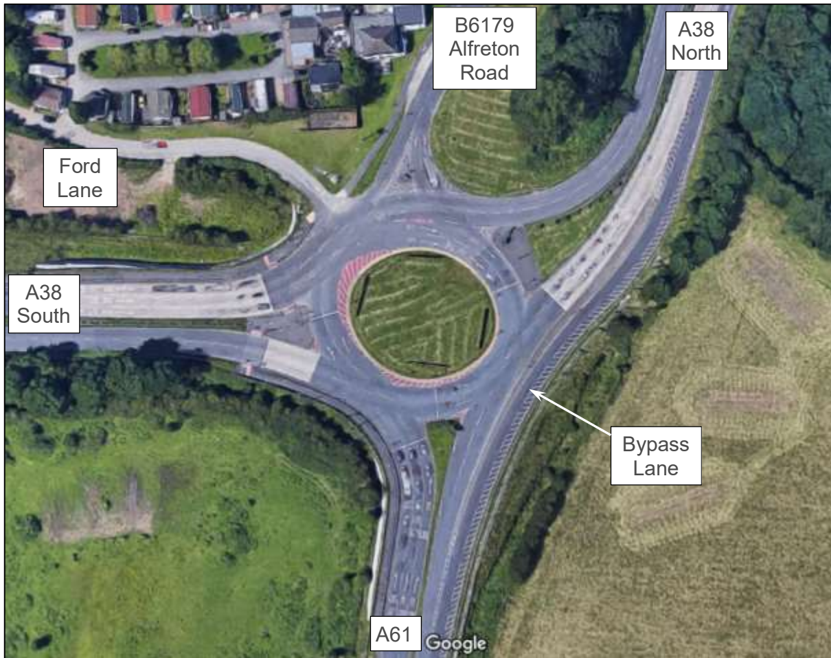
Figure 2.3: Little Eaton roundabout
